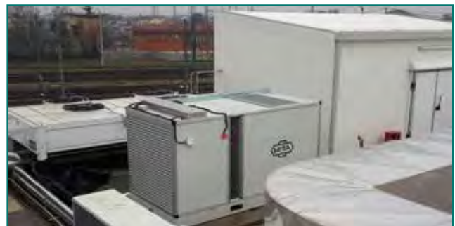
Alchemist in a refrigeration system
