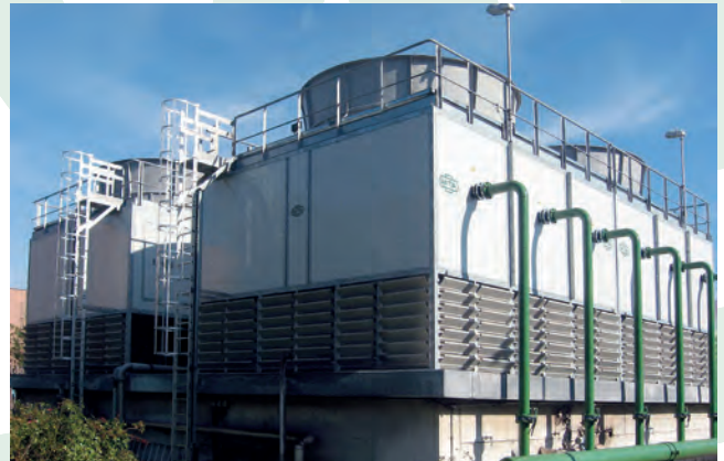
Plant after the replacement with MITA modules
