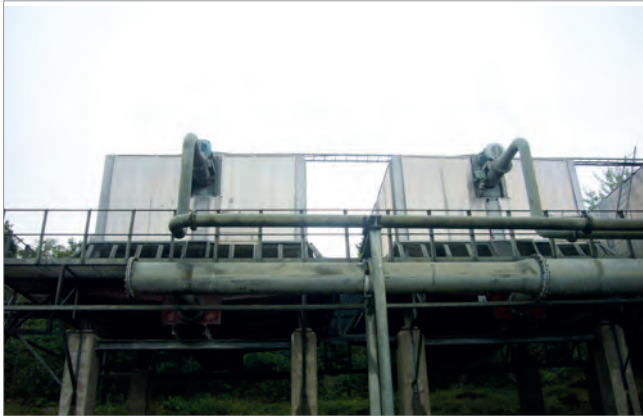
Plant before the replacement with a MITA solution
