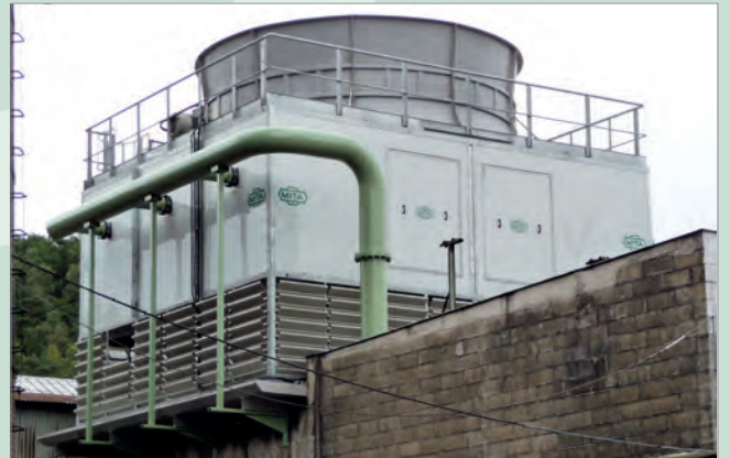
Plant after the replacement with MITA modules
