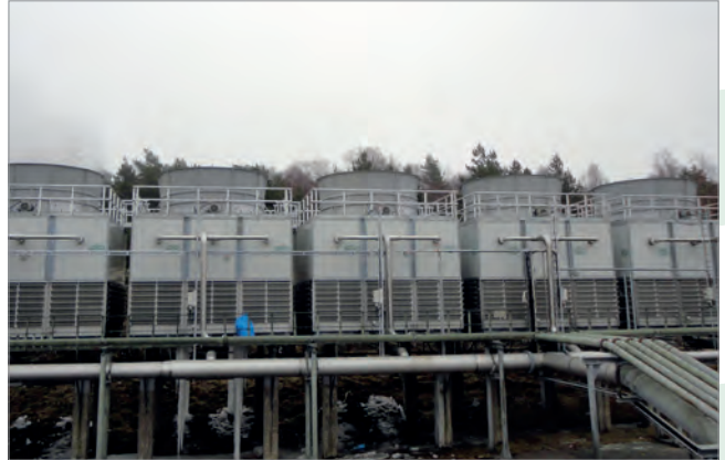
Plant after the replacement with MITA modules
