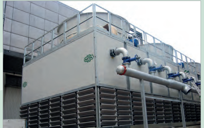
Plant after the replacement with MITA modules
