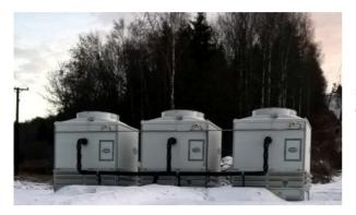
**Sweden**: No.3 units PME 2853 E CW SNOW, total cooling capacity 1.395 kW, towers complete with lower structure, louvers and basin.
