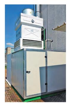
small/medium size cooling tower, which makes this solution the best one for limited thermal load plants.
