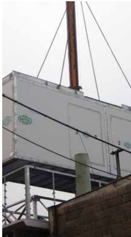
Handholding during installation.
