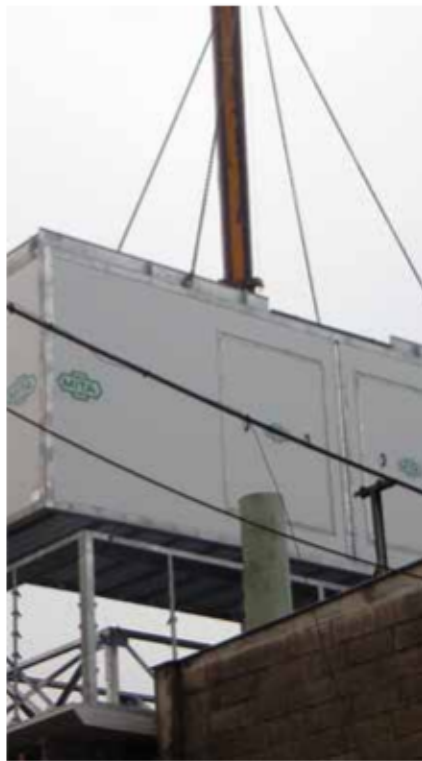
Handholding during installation.
