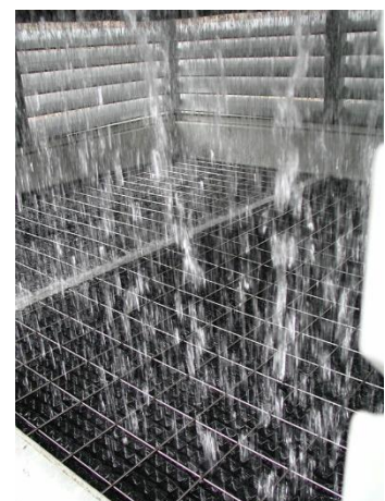
Sound absorbing mats over the basin's free surface
